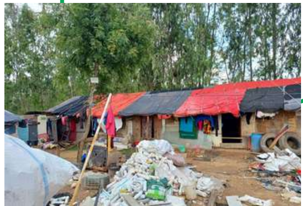
Situation at Shakthiman godown
