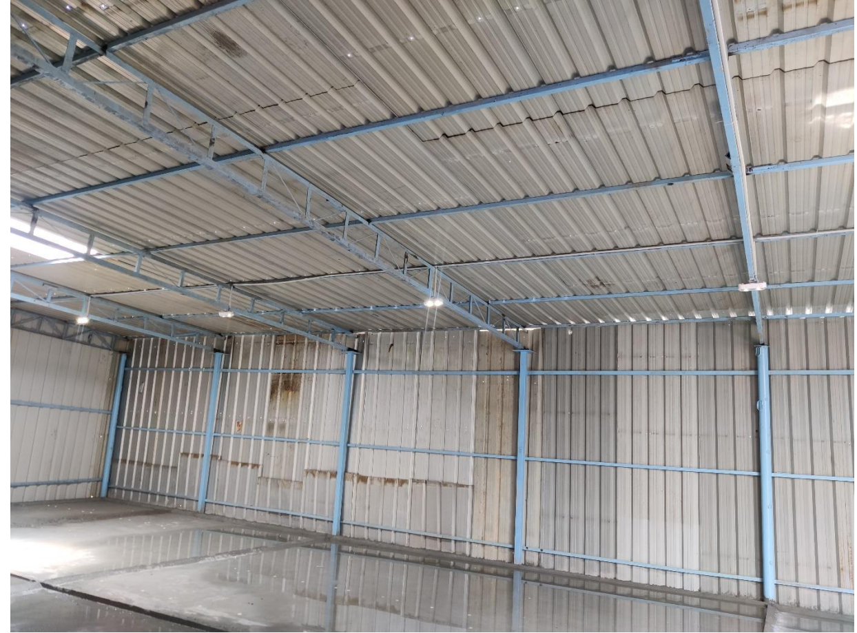
3 solar panels have been installed at the centre from SELCO India which will light up 6 lights and 3 charging points.
