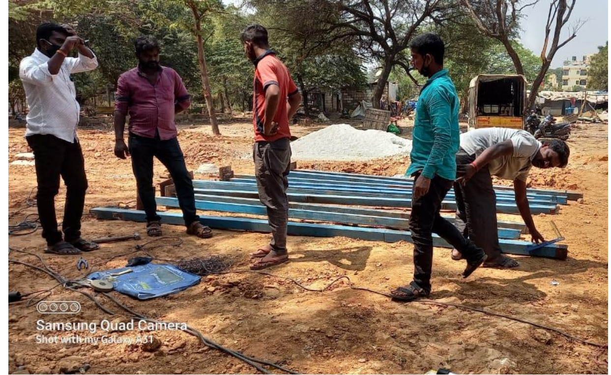
Fabrication work in progress
