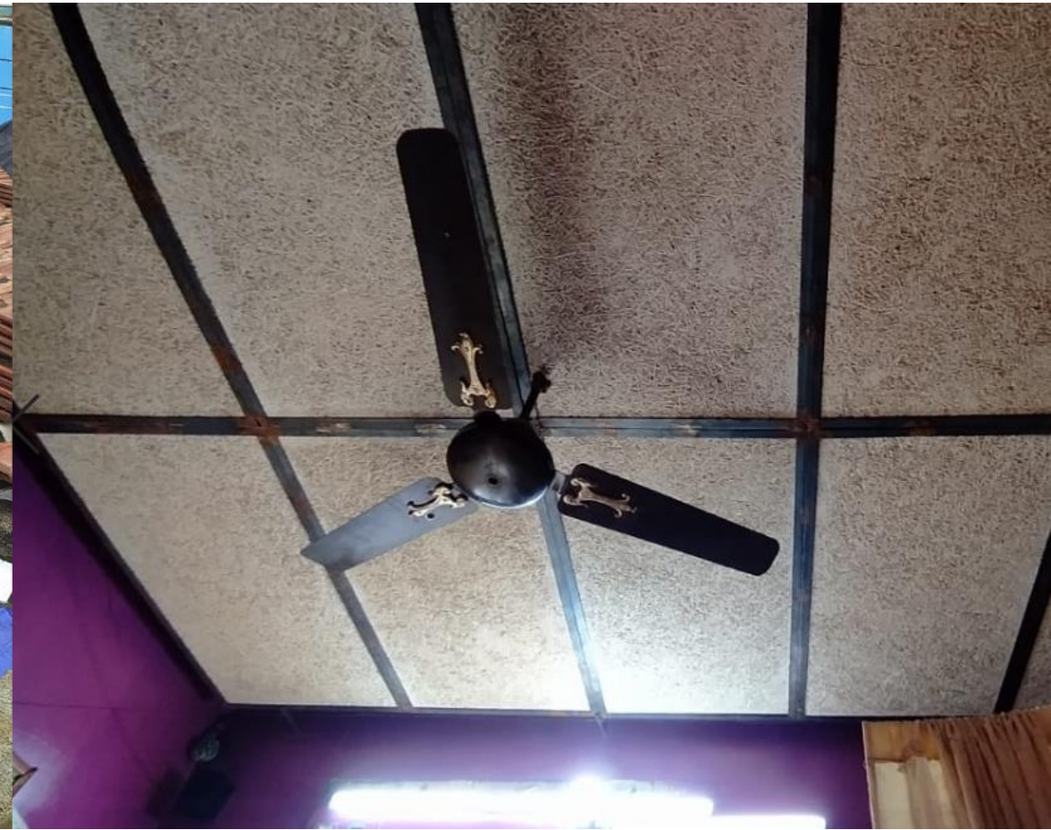
Wood Wool panels has been installed at Savitri's house
