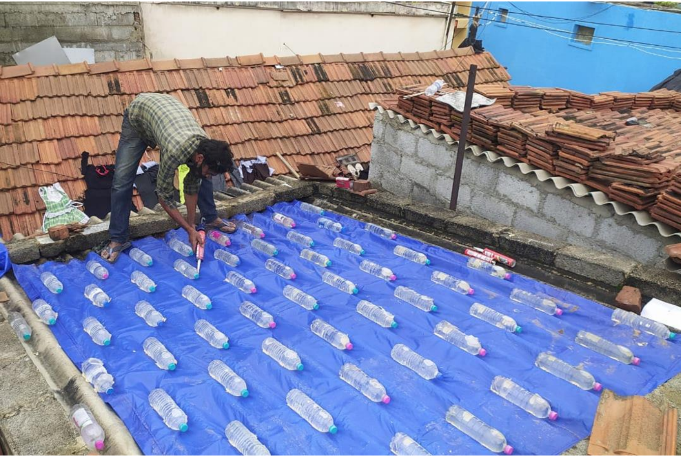
PET bottle solution was installed at Bugari: Children's library initiative by Hasiru Dala
