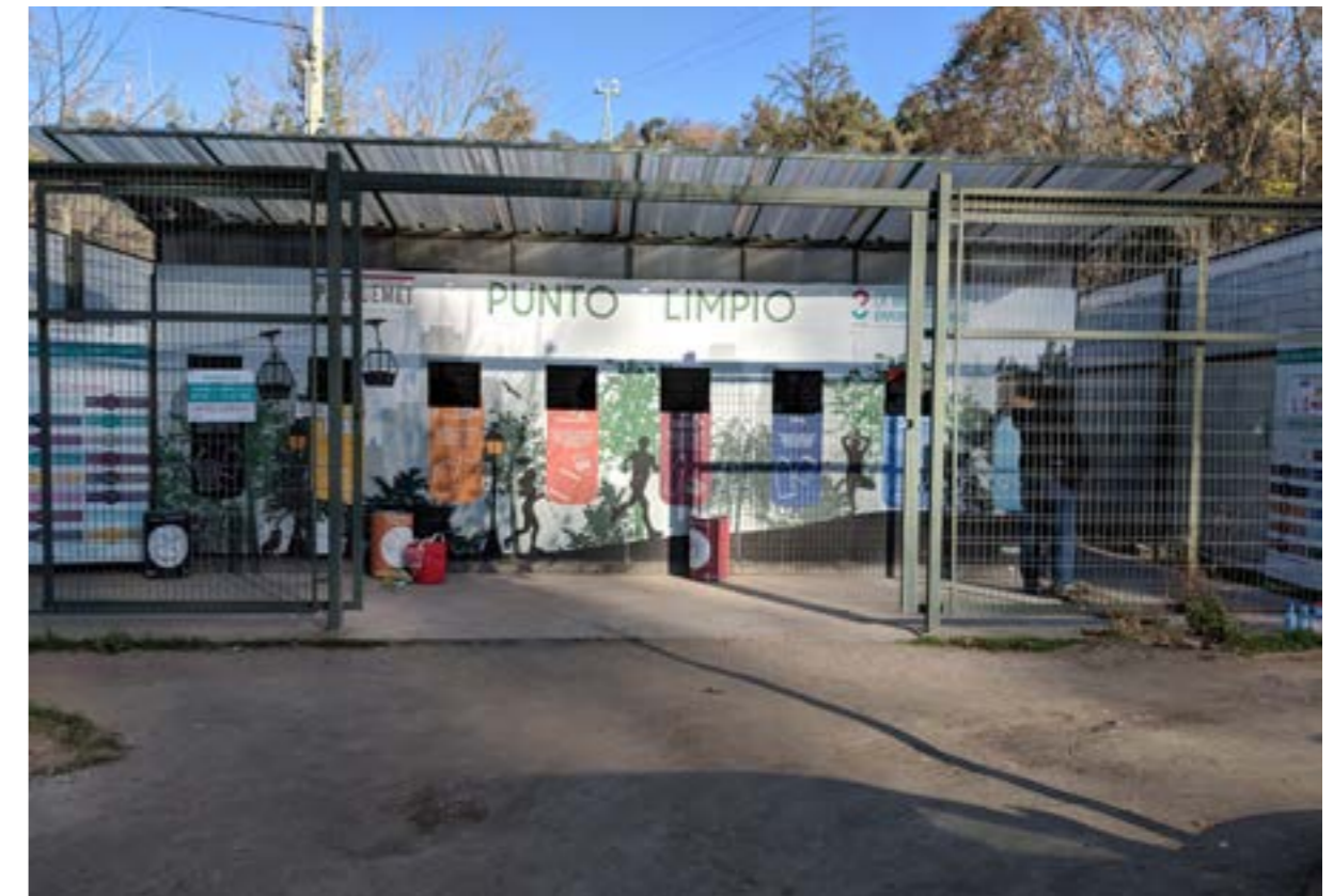
Exhibit 15: TriCiclos Clean Point facility
